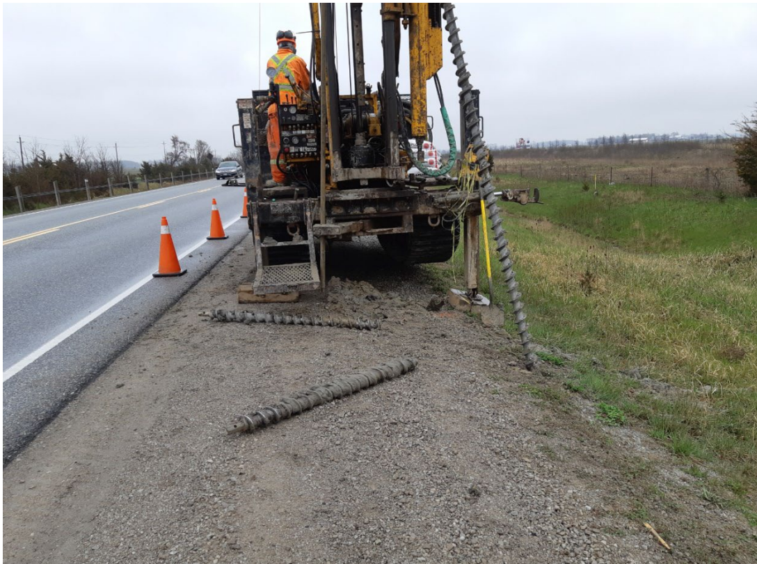
Photo 7 – Drilling at BH-20-07 – Culvert No. 06X-423/C0 – Hwy 3, 220 m East of Concession Road 8
