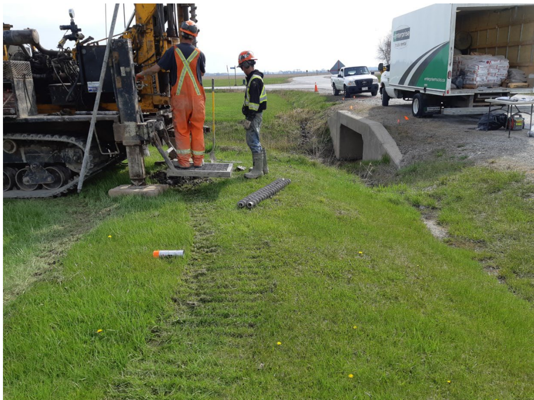
Photo 6 – Drilling at BH-20-06 – Culvert No. 06X-422/C0
