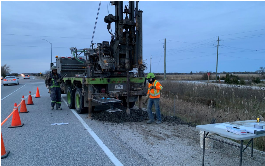
Photo 12 – Drilling at BH-21-02 – Culvert No. 06X-426/C0 North Extension– Hwy 3 Shoulder
