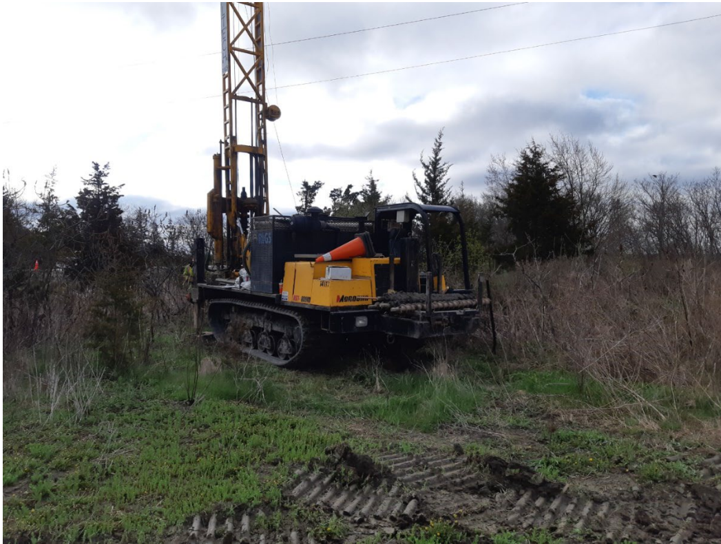
Photo 13 – Drilling at BH-20-11 – Culvert No. 06X-427/C0 – Hwy 3, 700 m east of County Road 27
