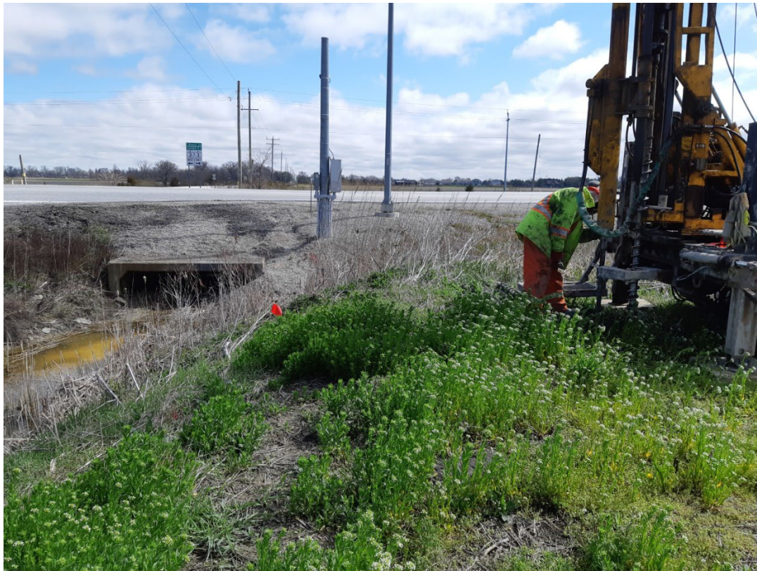
Photo 11 – Drilling Set up at BH-20-10 – Culvert No. 06X-426/C0 – Hwy 3 between County Road 27
