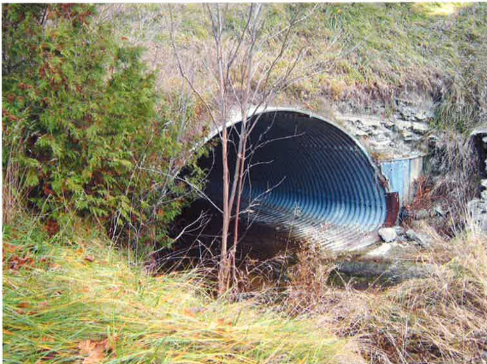
Photo 2 – Looking at CSP arch culvert inlet.
