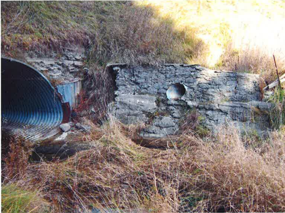
Photo 3 – View looking at retaining wall and drainage pipe on east side of inlet to culvert
