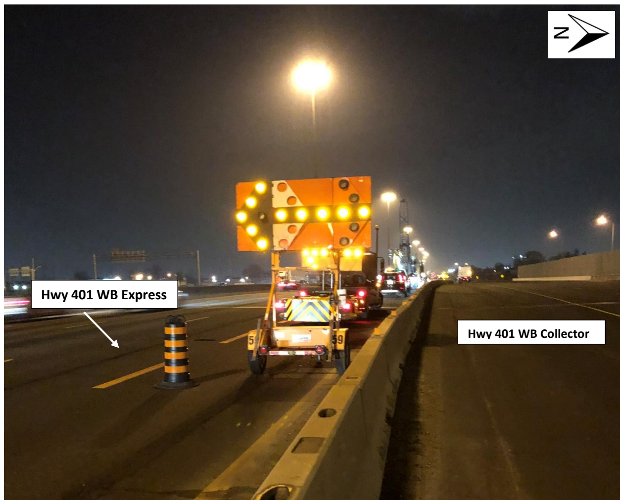
Photo C2-1: Looking towards West at Dufferin street Overpass on Highway 401 WB Express. – Traffic Control Set-up (November 2019)
