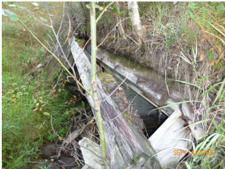
Figure 2.3 Culvert in poor condition (looking north)
