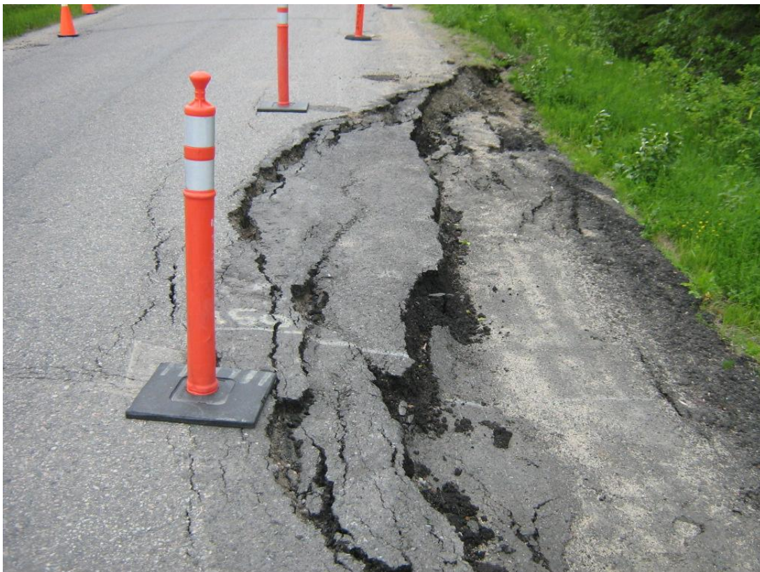
Figure 2.1 Slope Failure (looking north)
