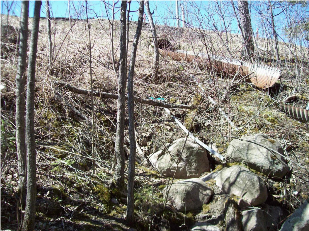
Figure 2.6 Cobble and boulder fill on foreslope (looking west)
