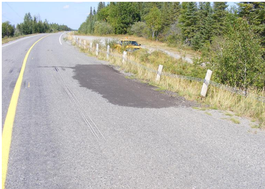
Photo 3: Looking Northerly (Culverts are located under the Patch)
