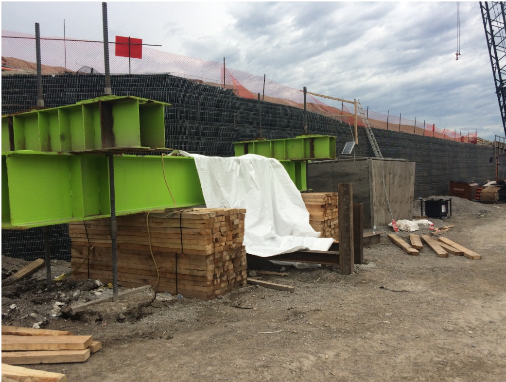
Photograph 2: Static load test reaction frame set-up
