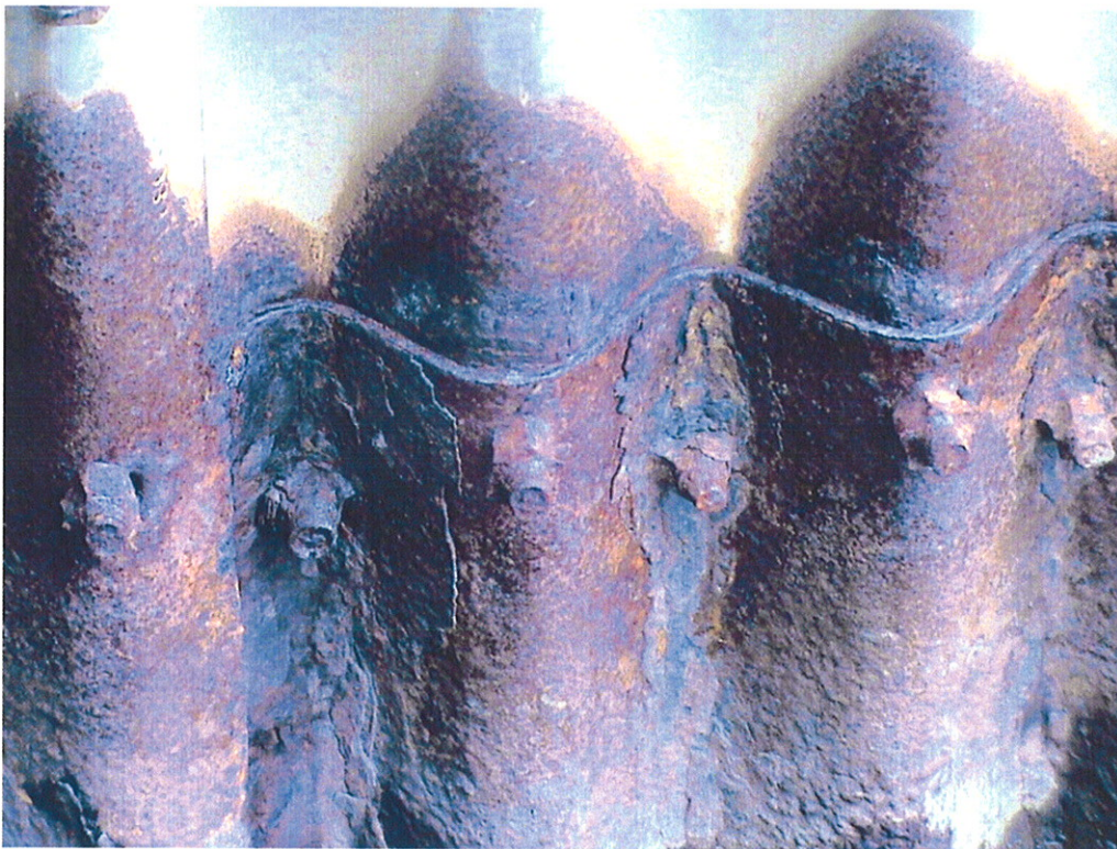
Photograph 4. Detail of Corrosion at Water Line
