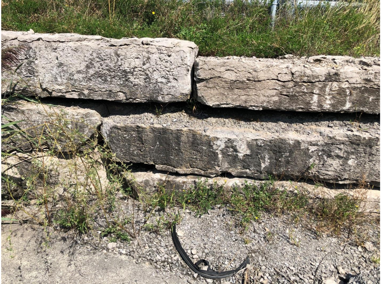
Photograph 2: Existing retaining wall structure looking southeast. The wall is currently acting as the existing culvert headwall. (September 3, 2019)
