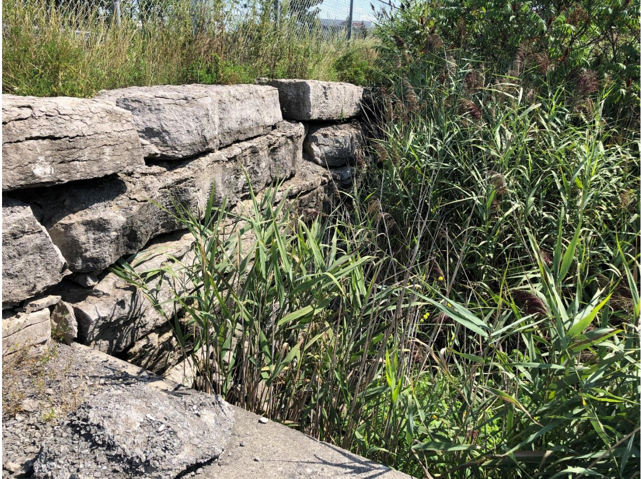
Photograph 1: Existing retaining wall structure looking south. The slope face at wall toe was covered with shrubs, sign of erosion on the slope face was not observed. (September 3, 2019)
