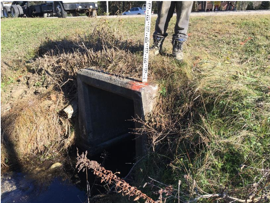
Photo 8: TBM location at top of culvert at outlet location
