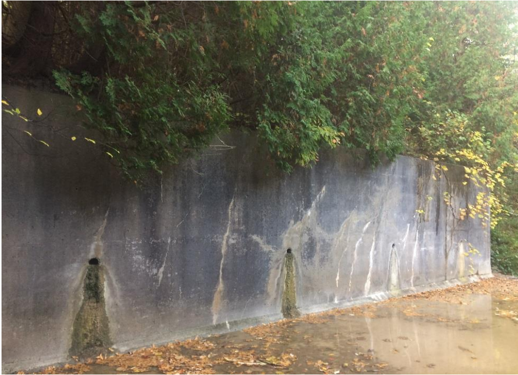
Photo 7: Heyrock Creek Culvert Outlet – – South Side Wing Wall
