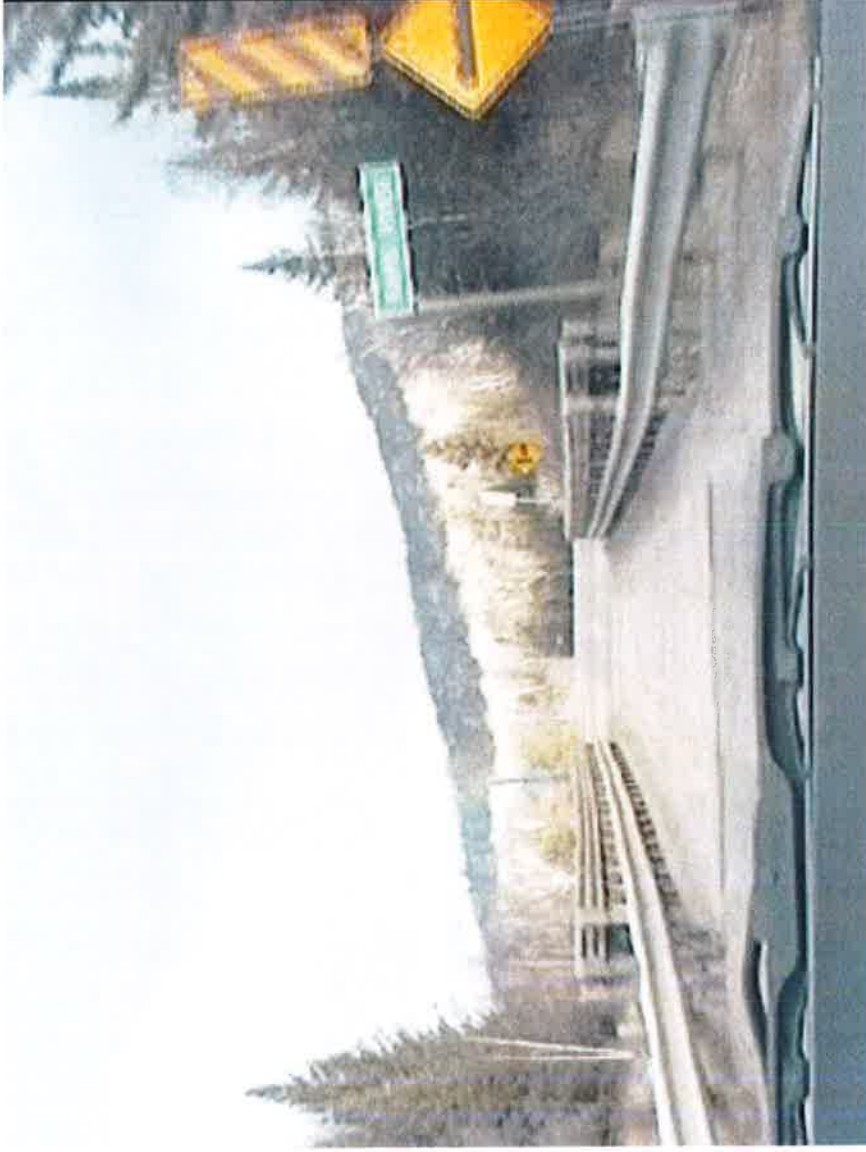
Photograph C-9 Single lane bailey bridge over Rapid River, Hwy 129
