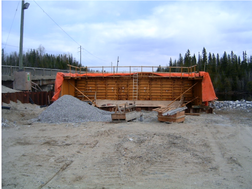
Photograph 1: Kabinakagami River Bridge. On south side of Highway 11, west bank of River, looking east towards the river. West side of the failed cofferdam and the formwork for West Abutment.
