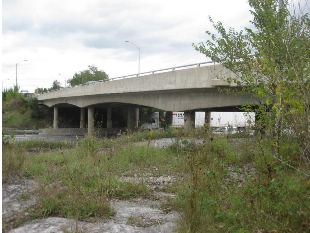
Photograph 1 – West side of existing bridge, looking northeast near new south abutment; note exposed bedrock surface
