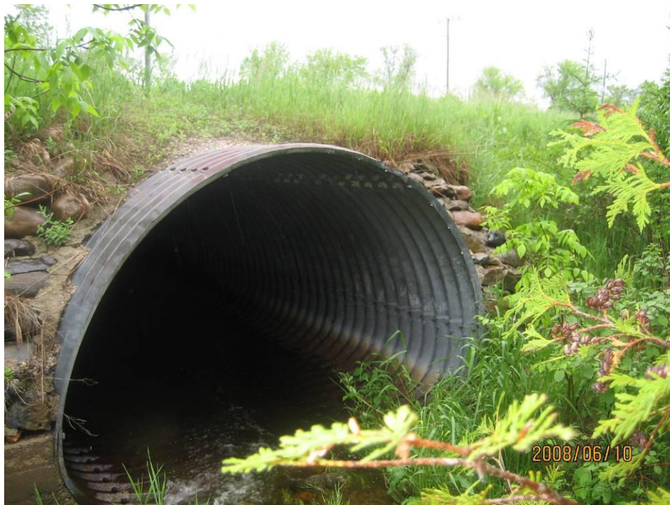
Figure 2.2 Minor erosion and loss of embankment (looking north)
