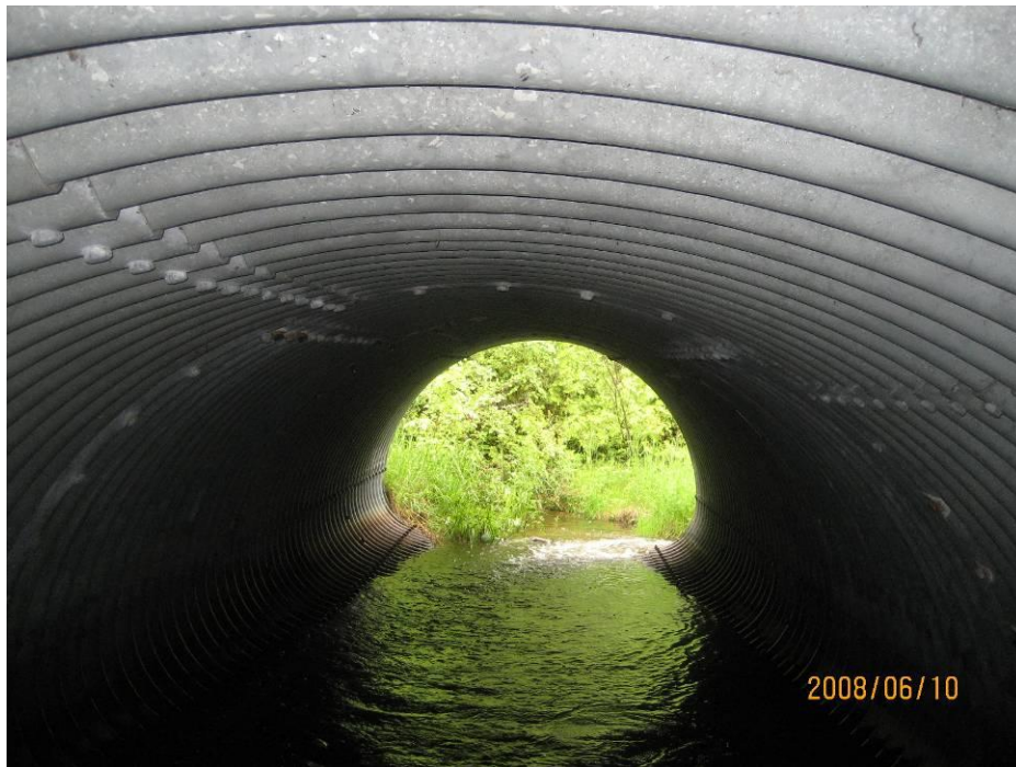
Figure 2.1 Corrugated Steel Pipe (CSP) culvert (looking south)
