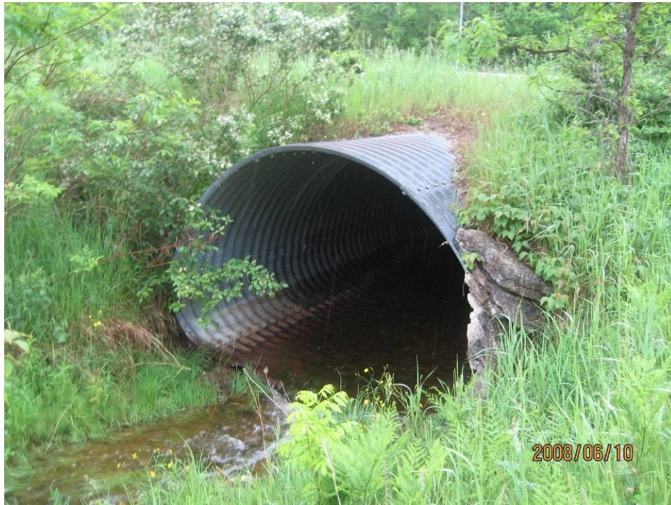
Figure 2.3 Outlet of the existing culvert (looking west)
