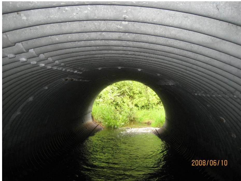
Figure 2.1 Corrugated Steel Pipe (CSP) culvert (looking south)
