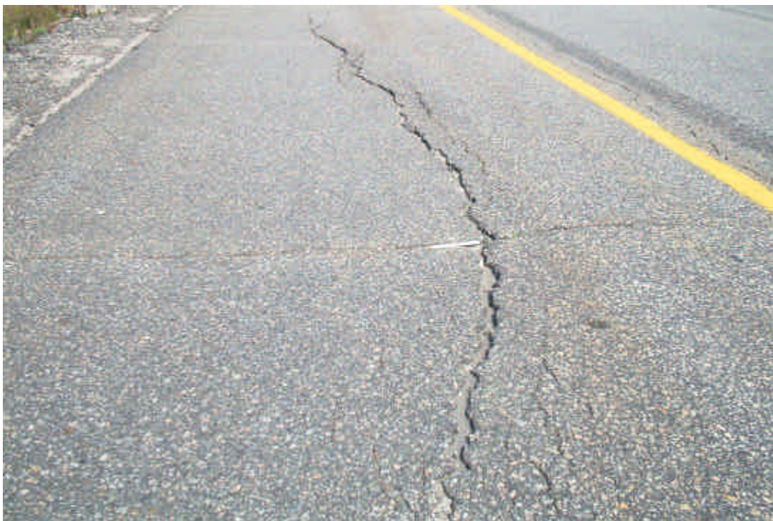
Photograph I-6 Cracks on Left Shoulder
