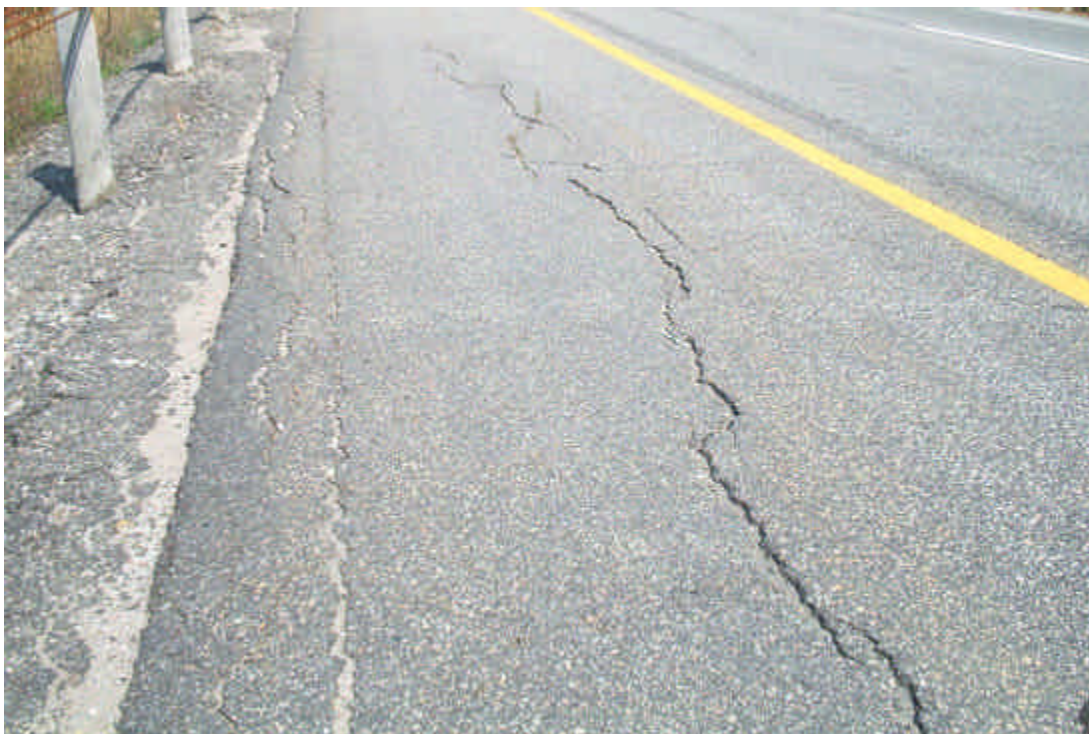
Photograph I-8 Cracks on Left Shoulder
