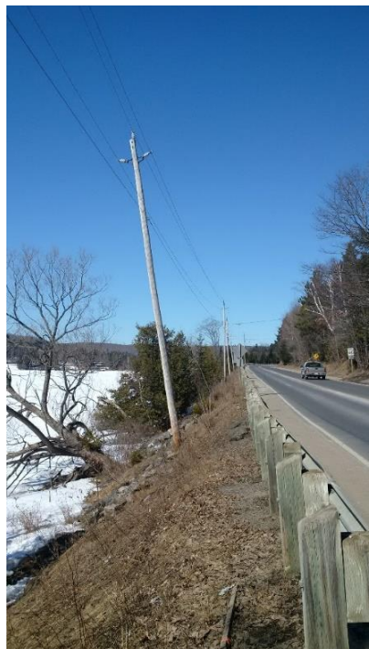
Photo 7: Area 2/3 – Highway 118 Looking North - Tilted Hydro Pole on Slope
