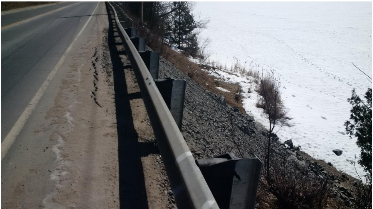
Photo 5: Area 2 – Looking South – Longitudinal Crack and Sagging Guardrail
