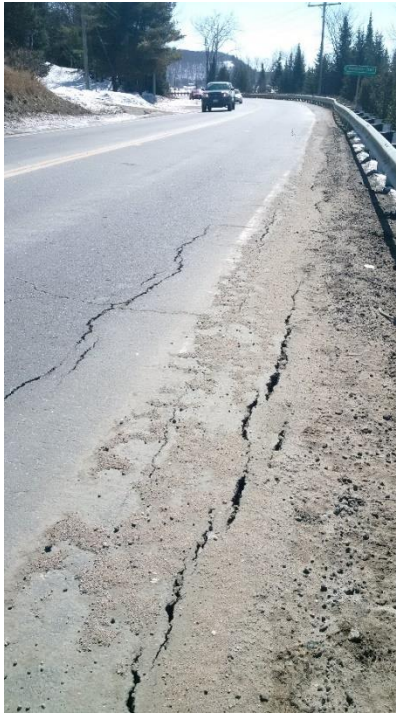
Photo 4: Area 1 – Highway 118 Looking South – Longitudinal Cracks on Shoulder
