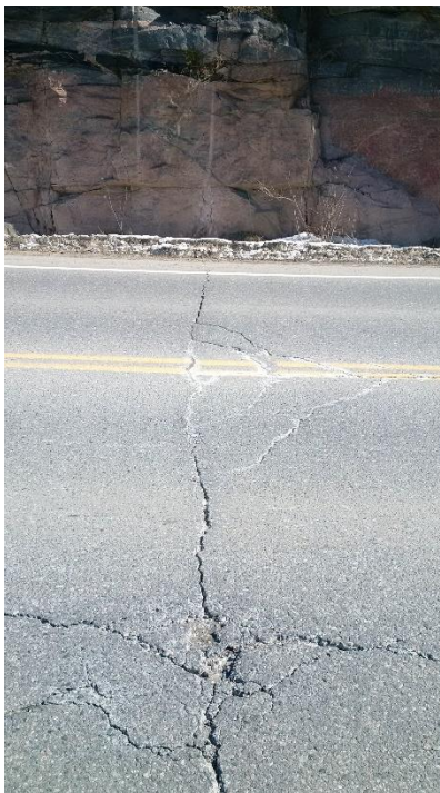
Photo 3: Area 1 – Looking East – Transverse Cracks (Rock Cut in Background)
