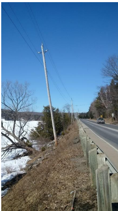
Photo 7: Area 2/3 – Highway 118 Looking North - Tilted Hydro Pole on Slope
