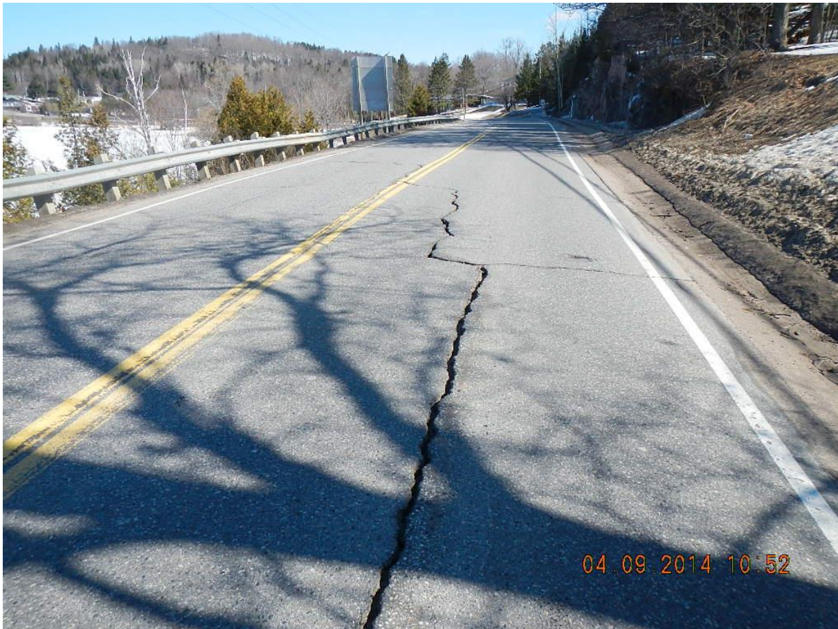
Photo 1: Area 1 – Highway 118 Looking North Significant Tension Cracks traversing entire roadway (April 2014) (Courtesy of AECOM)
