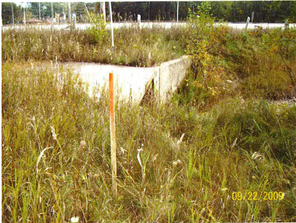
Photograph 1. Retaining wall at the existing culvert inlet and embankment
