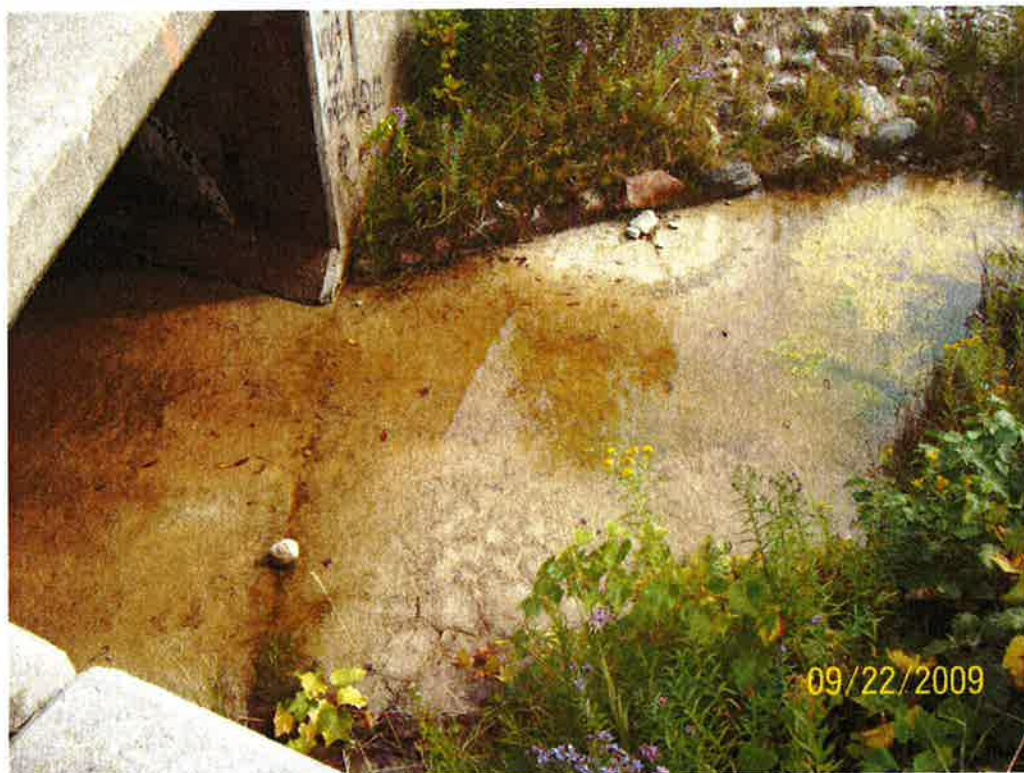
Photograph 2. Existing culvert inlet and concrete slab
