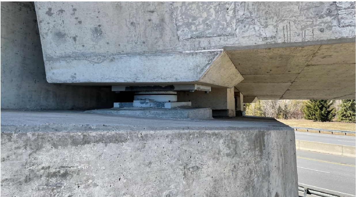
Photo 6. Looking west at south abutment bearings. (2021/03/29)
