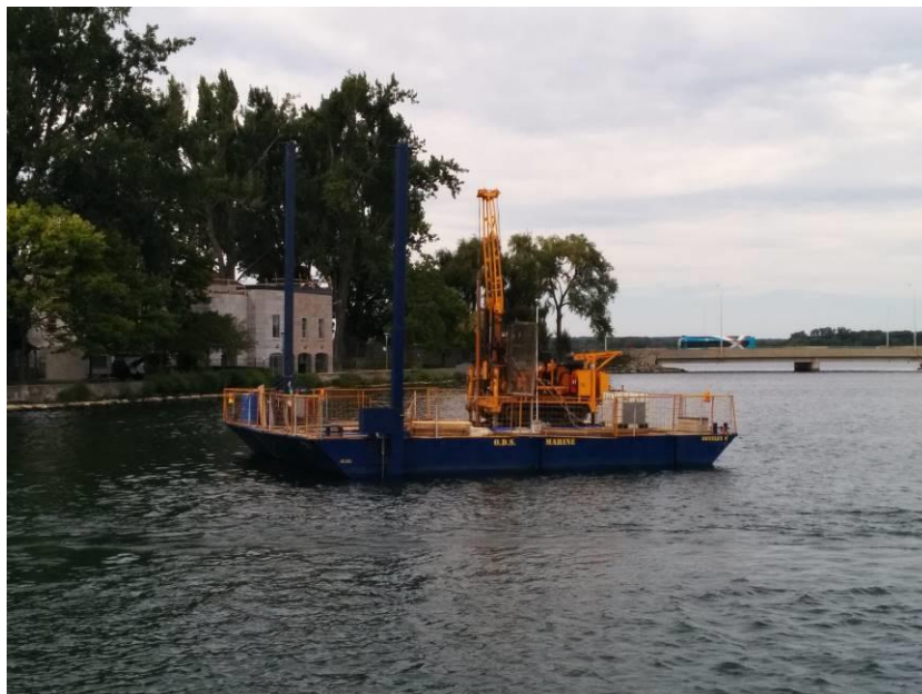
Photo 6. Barge Setup, Supported with Spuds, Near Barrack Terminal
