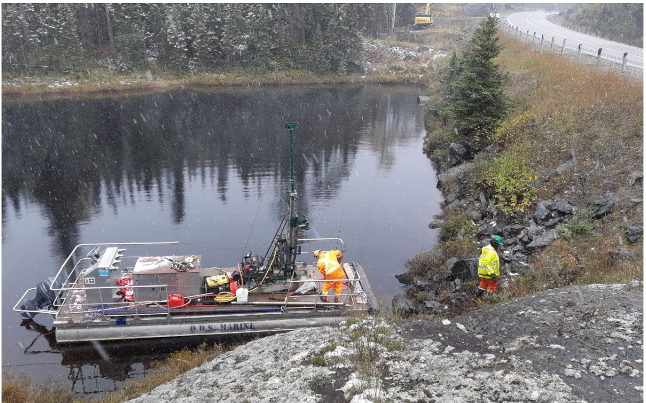
Photo 14 – Highway 17 - Area 4 – Drilling Setup at BH-19-4-01 – Looking East
