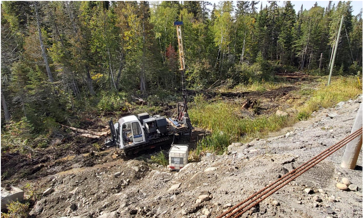
Photo 7 – Highway 17 - Area 1 – Drilling at BH-19-1-03 - Looking West
