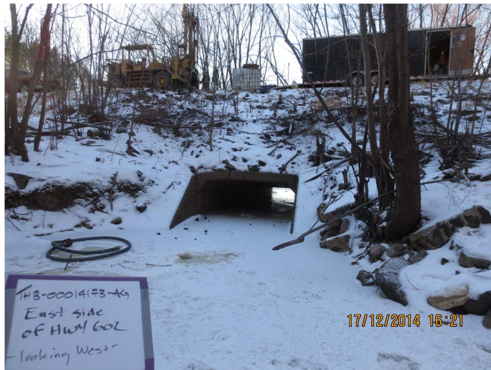
Photo 1. Inlet of existing culvert at east side of highway
