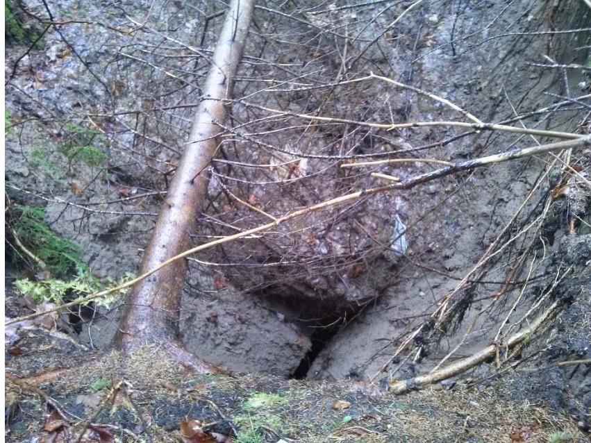
Photo 7: Erosion above inlet, indicating separation of culvert section
