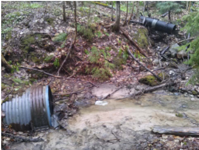
Photo 6: Outlet of southbound ditch culvert
