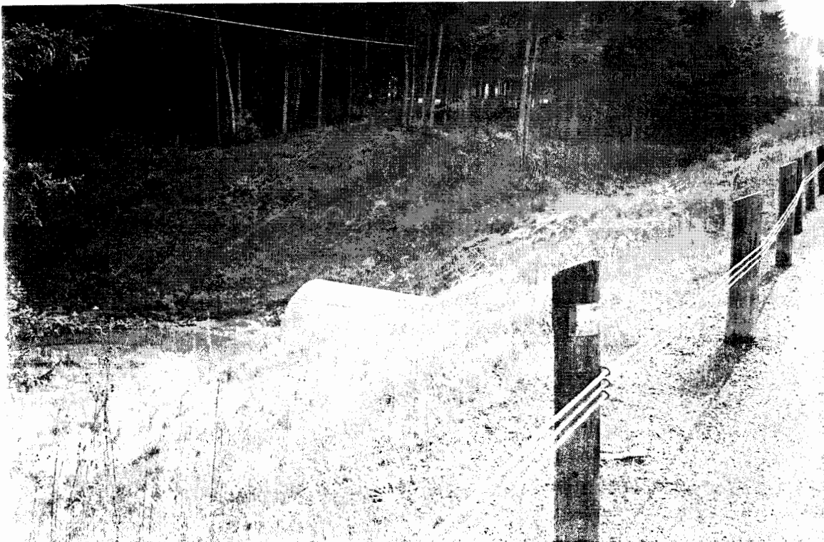
Photograph 2: ~Station 12+750 – Looking south east at the existing eastern embankment slope. (Note: The culvert outlet at the toe of the slope.)
