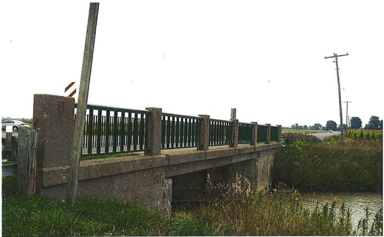
Photo No. 1c: Barrier Railing System for Concession #18 Drain Bridge
