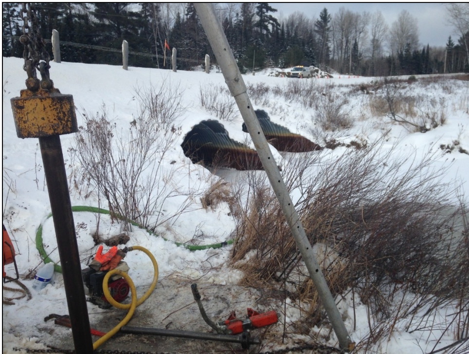
Photograph P2: Looking north from the south side of the Phillips Creek at the location of Borehole PC-4. Two existing CSP culverts are visible. (January 13, 2015)
