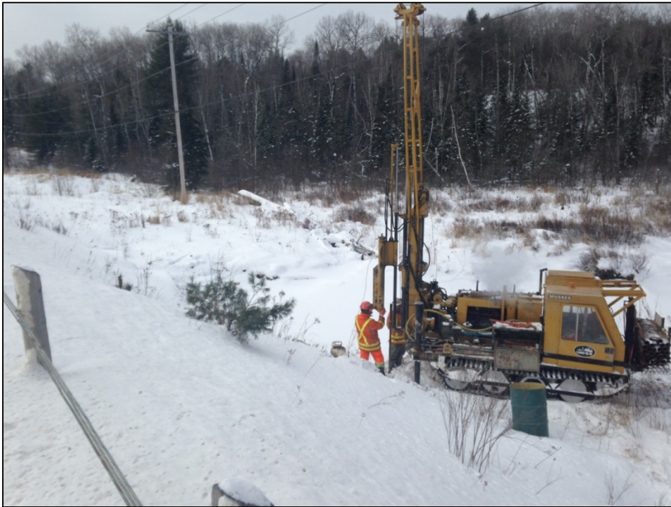
Photograph P3: Looking south west from Highway 129 northbound lane shoulder. Borehole PC-1 advanced by using a track mount at this location. (January 13, 2015)
