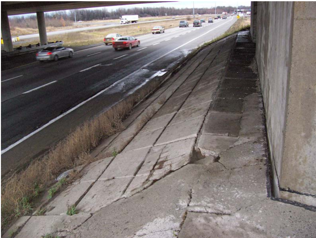
Photo 1: Looking east along slope paving. Note cracking and faulting.
