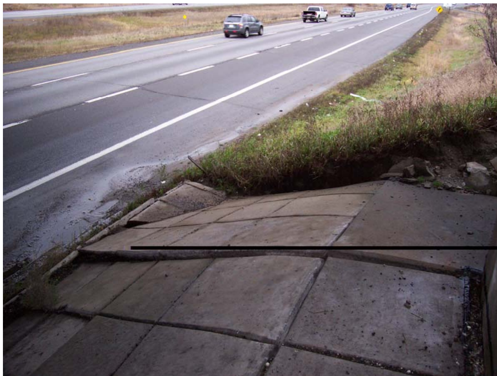
Photo 2: Erosion of soil at east edge of slope paving and resulting settlement and cracking of concrete.
