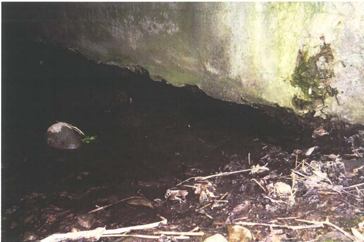
Photo No. 4: Culvert outlet with signs of erosion and deterioration at the south side.
