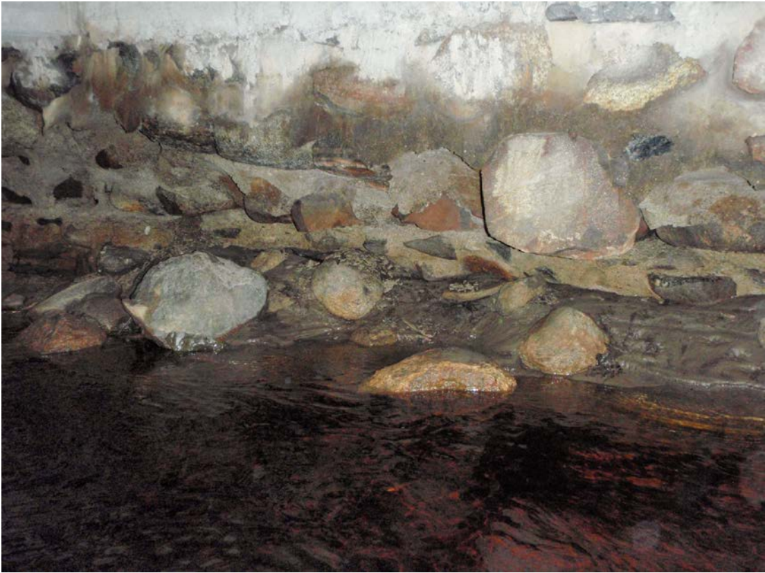
Photo No. 11: Deterioration of stone wall and concrete in middle-west section of culvert.
