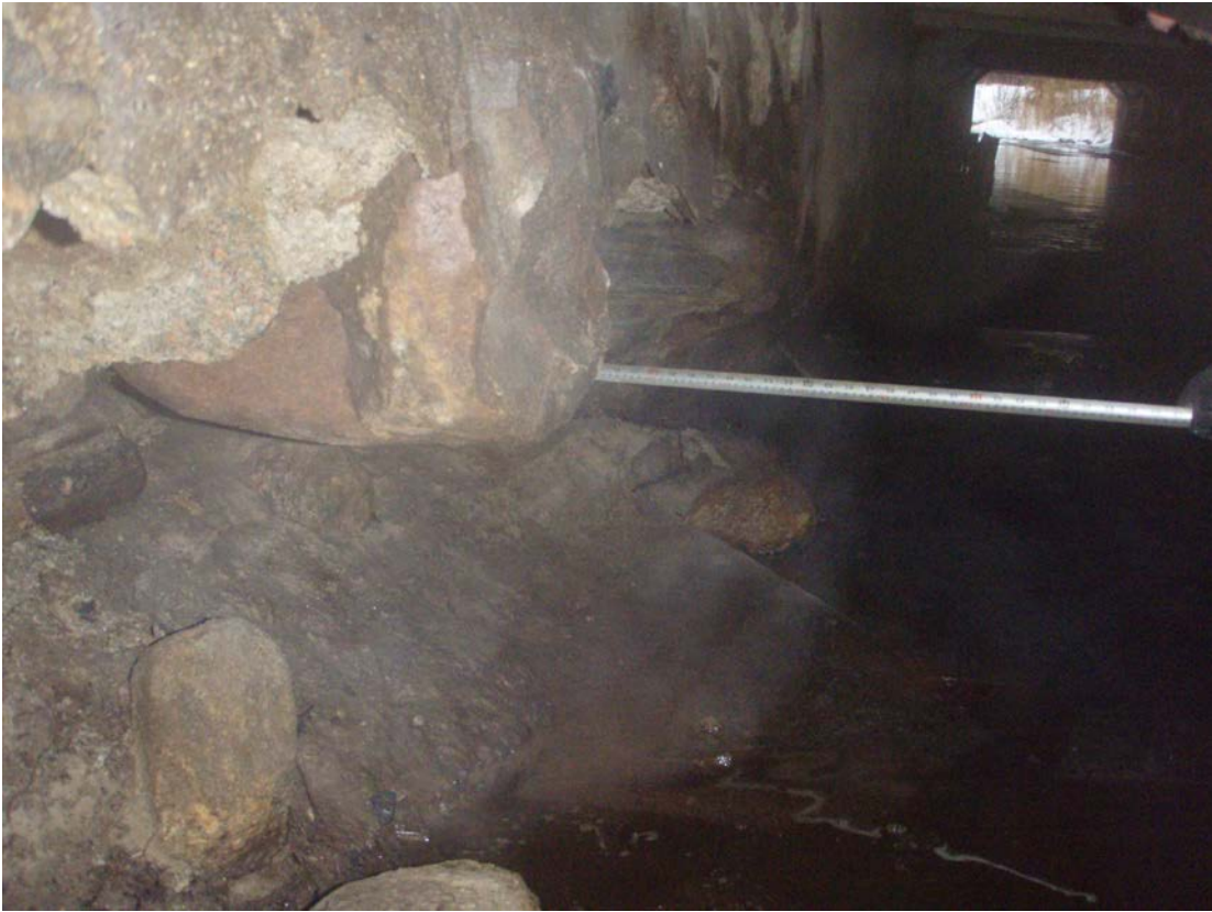
Photo No. 9: Deterioration of stone wall and concrete in middle-west section of culvert.
