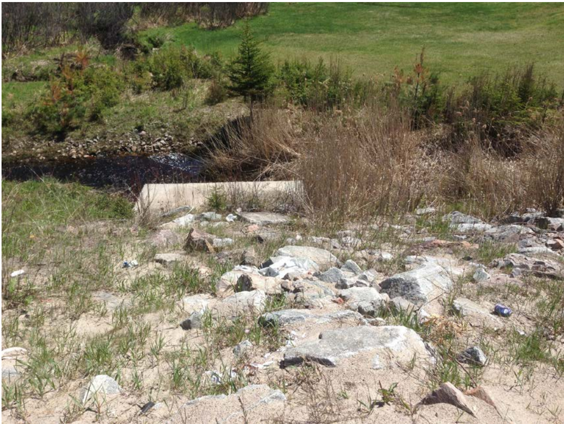
Photo No. 4: Culvert outlet, east side of Highway 11 showing rock fill on slope.
