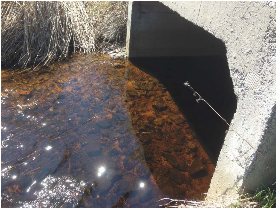
Photo No. 8: Culvert outlet, showing creek bed and sediment in culvert.
