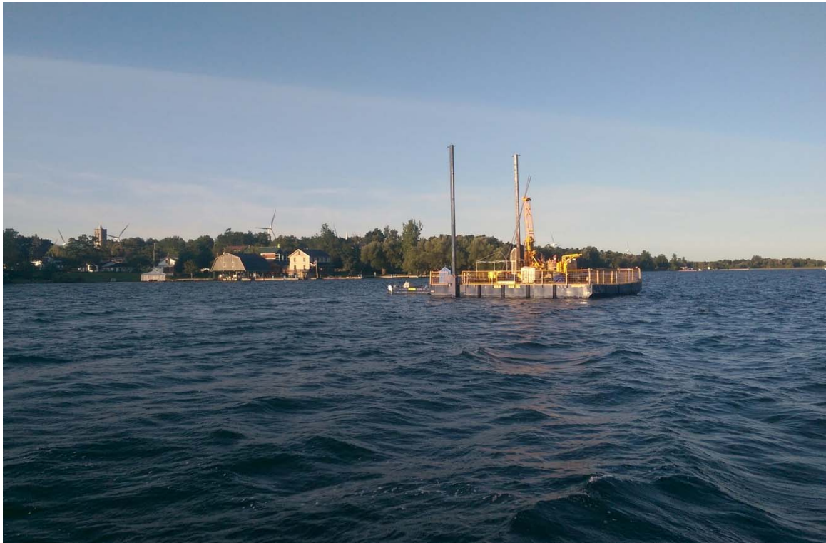
Photo 3. Barge Setup, Supported with Spuds, Near Marysville Terminal (taken July 2018)
