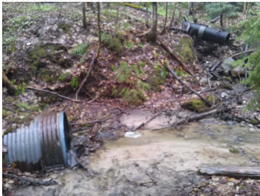
Photo 6: Outlet of southbound ditch culvert
