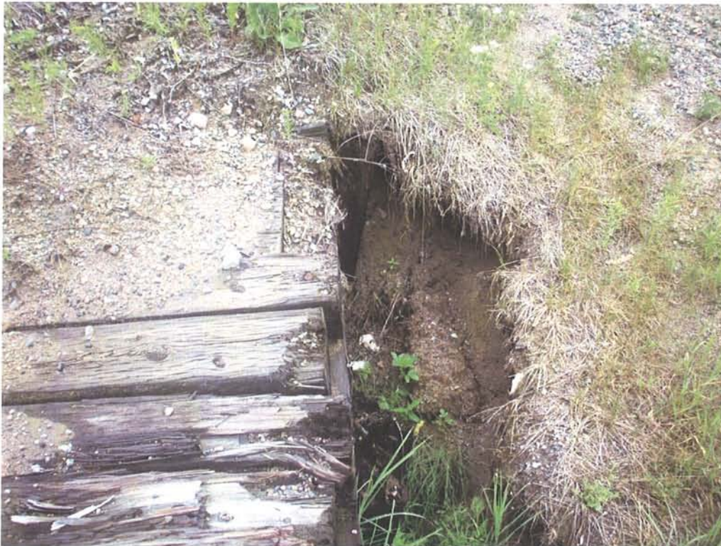
Photo No. B4: Site No. 46-398/c. Erosion at edge of culvert on south side.
