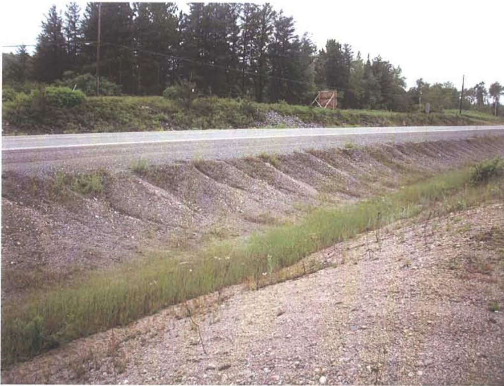
Photo No. B3: Site No. 46-398/c. Erosion of ditch slopes beside culvert.
