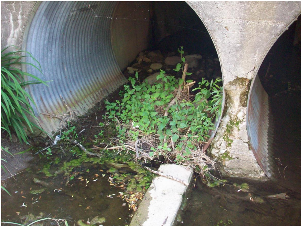
Photo No. 6: North end of culvert, east CSP with rock and tree debris.
