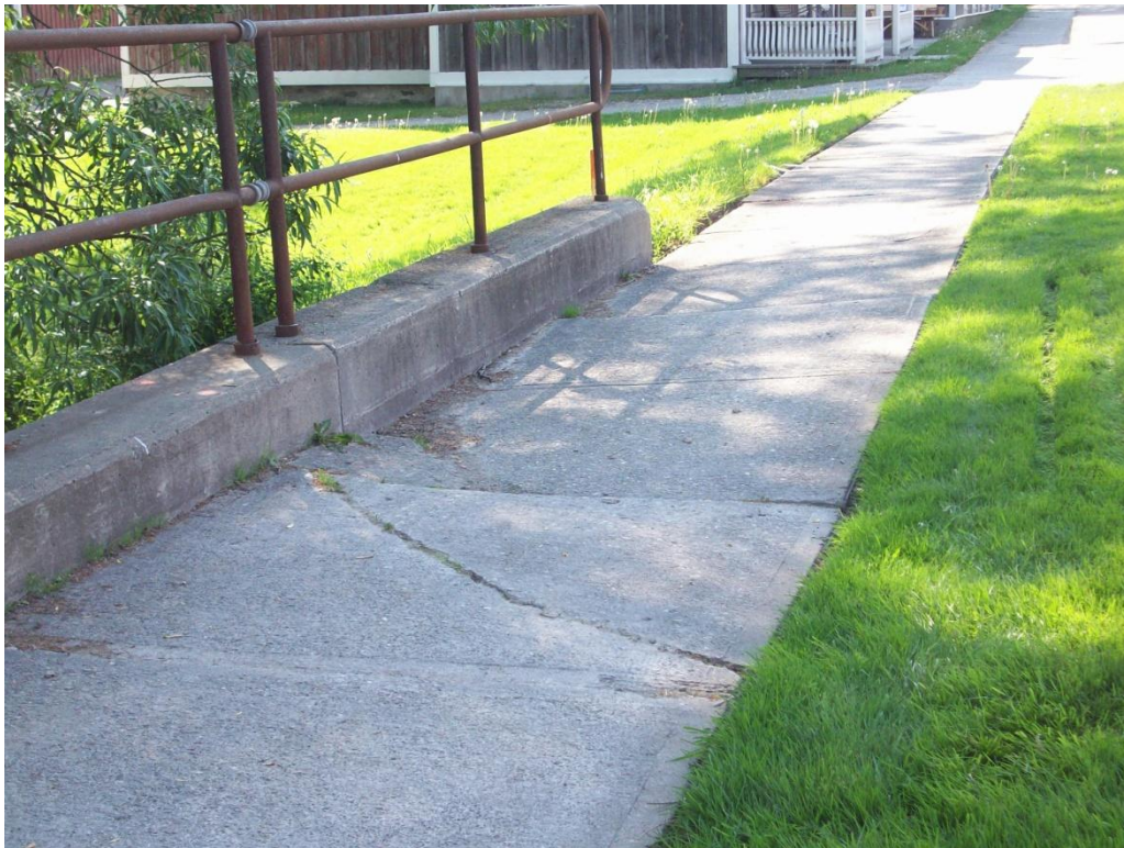
Photo No. 7: Settlement and cracking of sidewalk at south end of culvert.
