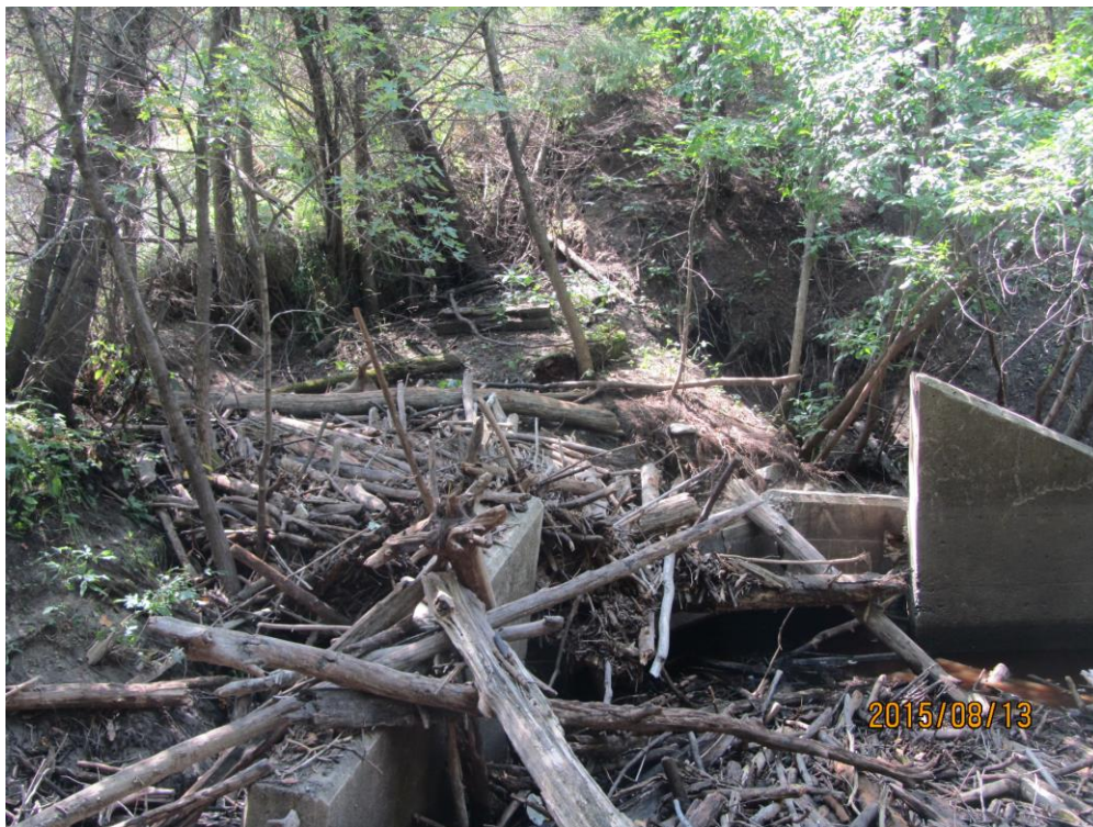
Photograph 4 – Debris, scour and erosion at the north end of the culvert
