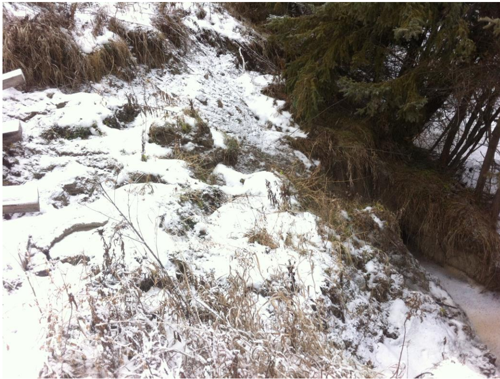
Photograph 6 – North embankment slope failure above the culvert location
