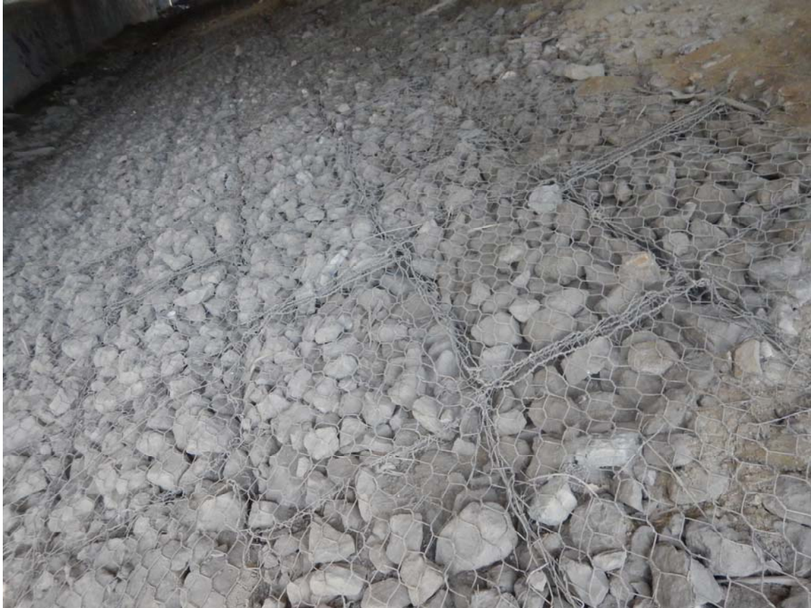
Photo 4: Gabion baskets at the lower portion of the west forward slopes between the existing EB collector bridge and EB express bridge, west side of Etobicoke Creek; looking south.
