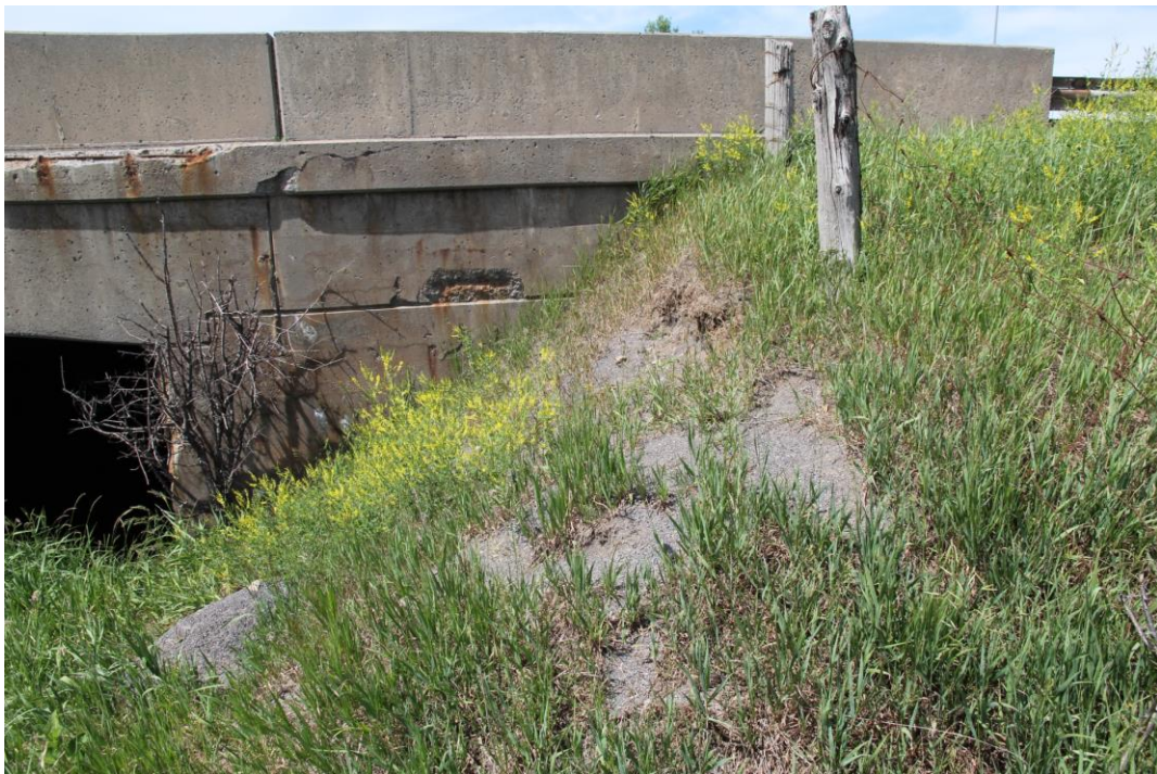
Photo 2 - Erosion at South East Approach Fill Due to Burrowing Animals
