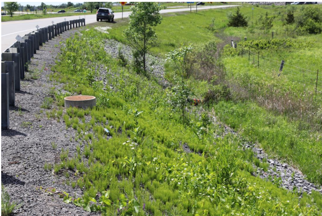
Photo 6 - Rock Lined Ditch at Toe of Slope, E-N Ramp
