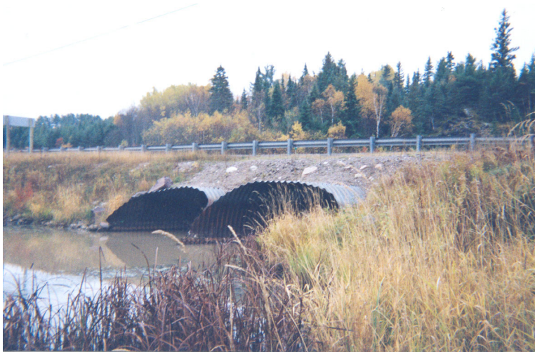
Photo 8 Twin CSP culverts through Highway 17. North end facing southeast.
