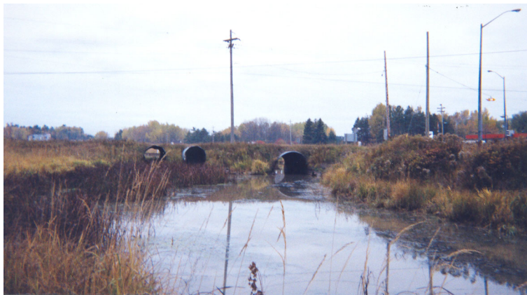
Photo 9 Single & Twin CSP culverts through Lake Huron Dr. South East end facing west
