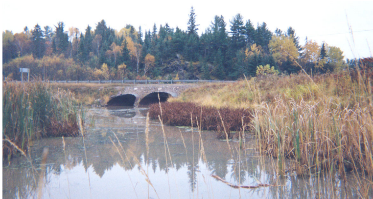
Photo 7 Twin CSP culverts through Highway 17. North end facing south.
