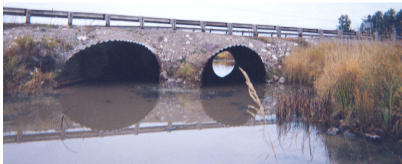
Photo 6 Proposed gabion basket retaining wall Location: East of Lake Huron Dr., facing North. Twin CSP culverts through Highway 17. South end facing north.
