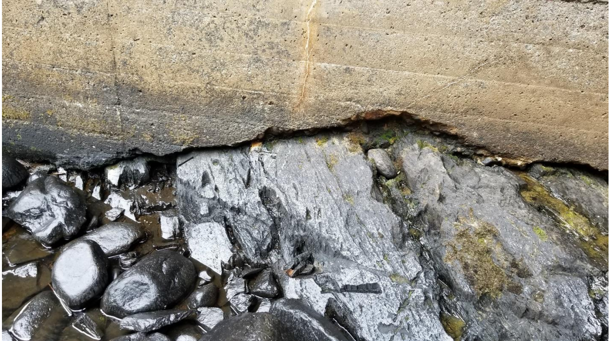
Photo 5: Voids beneath east footing near north end (Taken: August 27, 2017)
