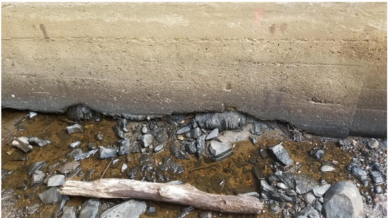
Photo 6: Voids beneath east footing near south end (Taken: August 27, 2017)
