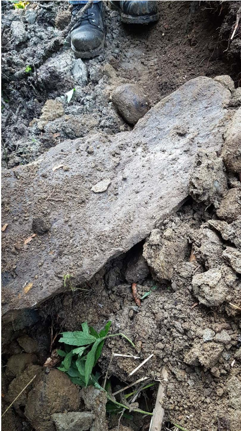
*Photograph 4: Boulder encountered while excavating TP 18-109B*
