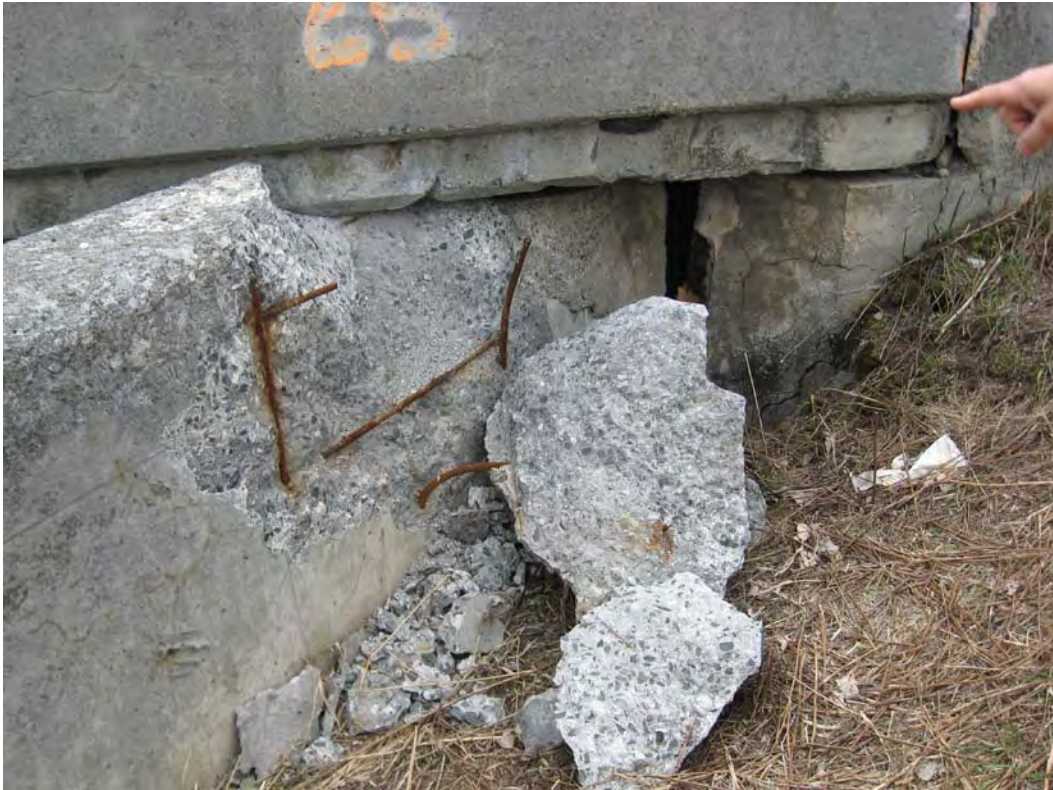
Plate 3 – Retaining wall contact with EBL and associated damage
