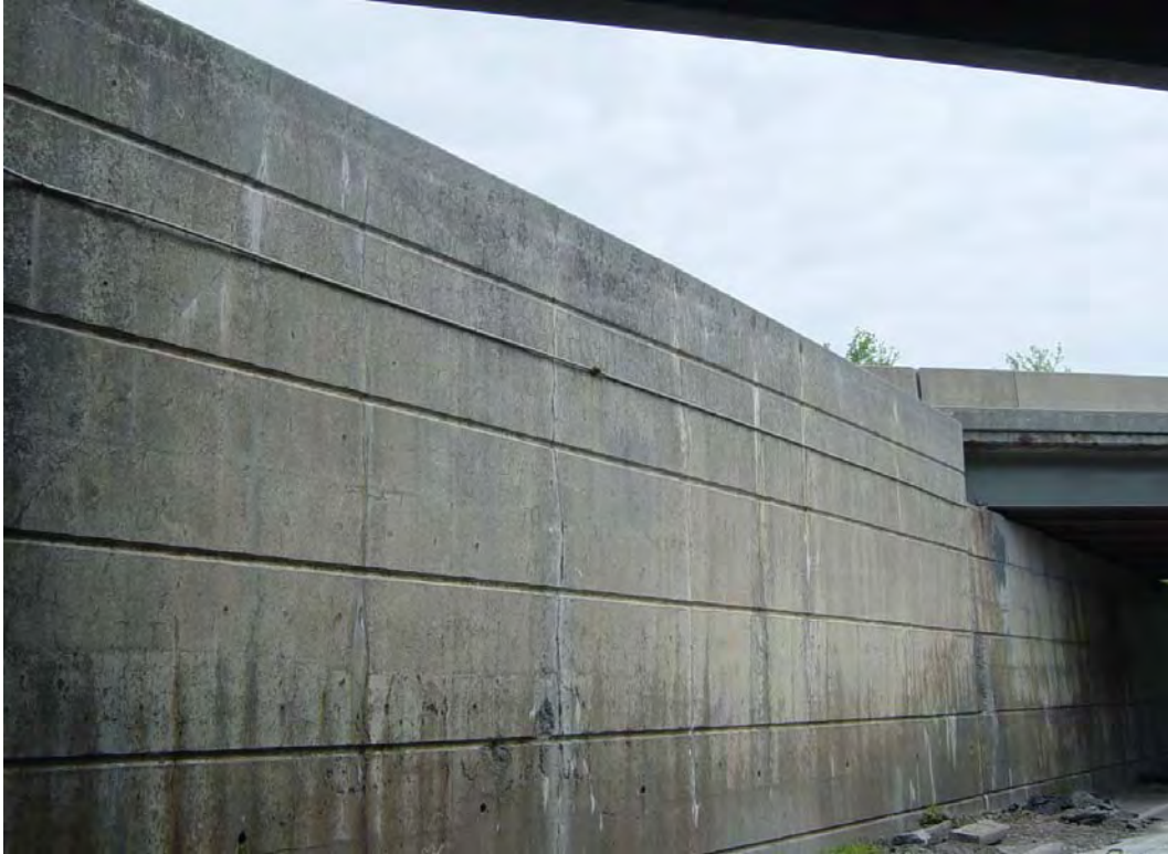
Plate 5 – Vertical cracks in median retaining wall
