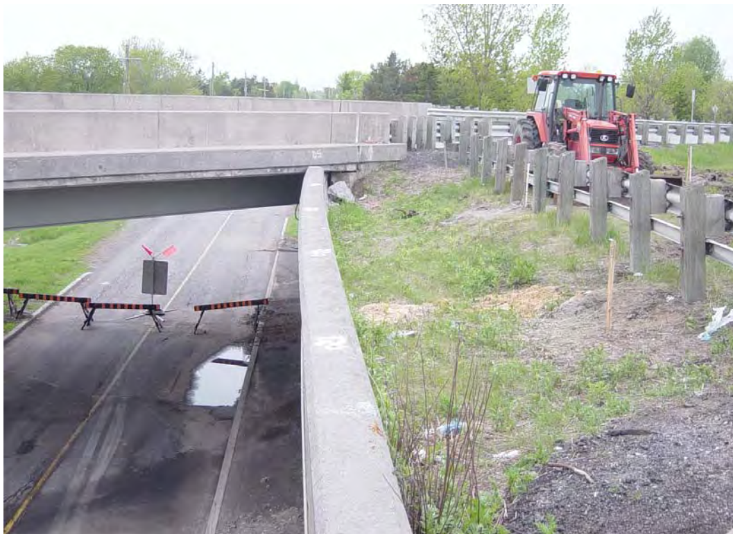
Plate 4 – Median retaining wall distress (facing south)
