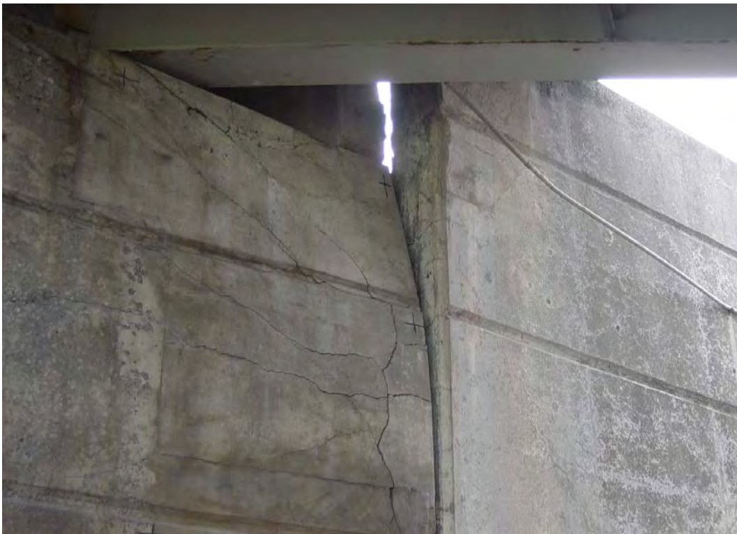
Plate 6 – Distress at EBL abutment and median retaining wall
