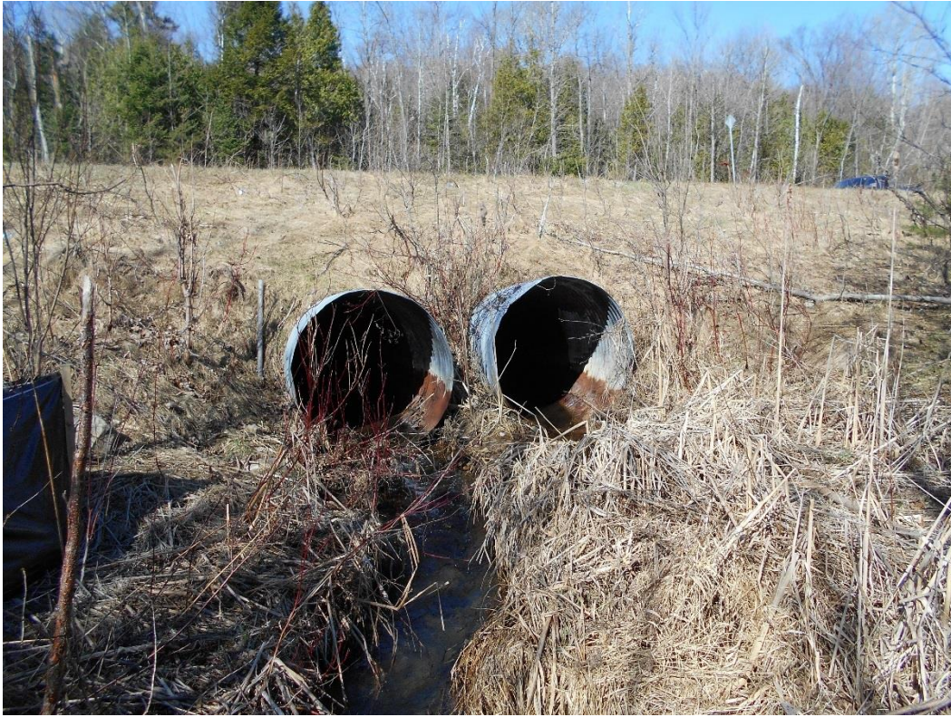
Figure 3: Existing condition of culverts and embankment at outlet
