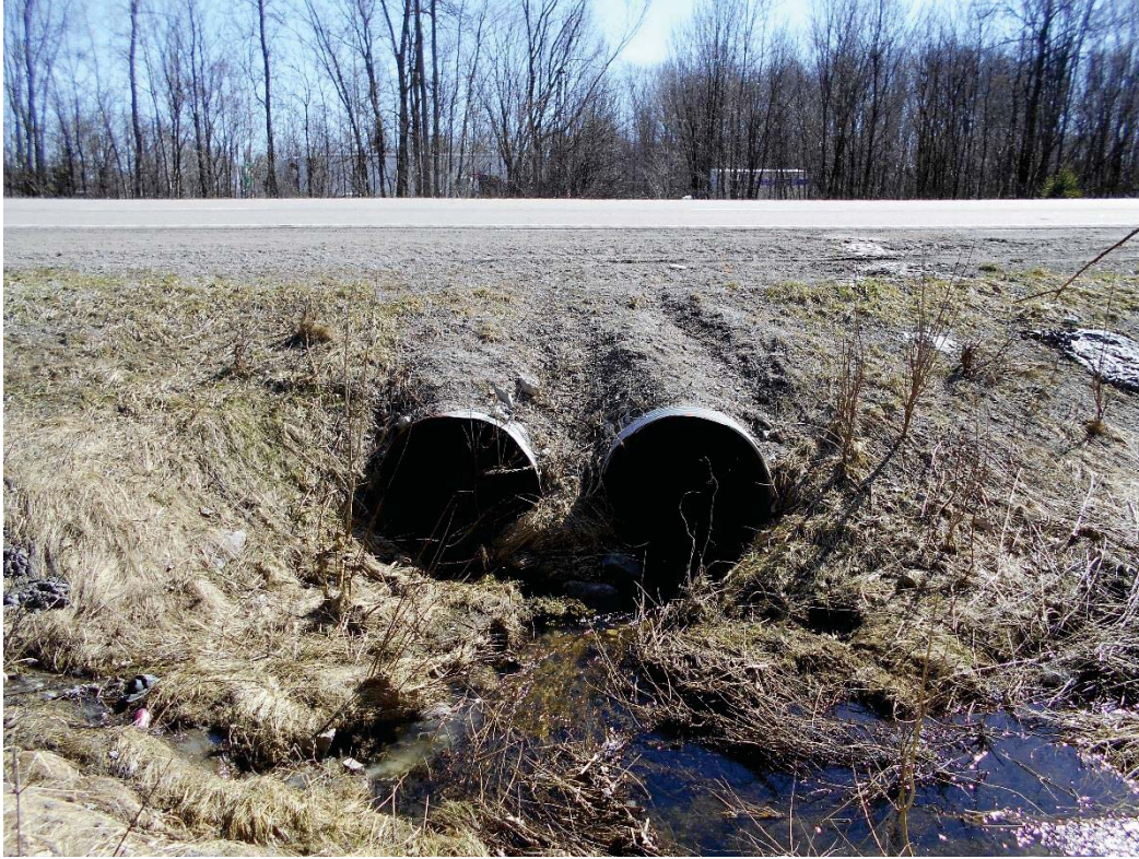
Figure 5: Existing condition of culverts and embankment at inlet
