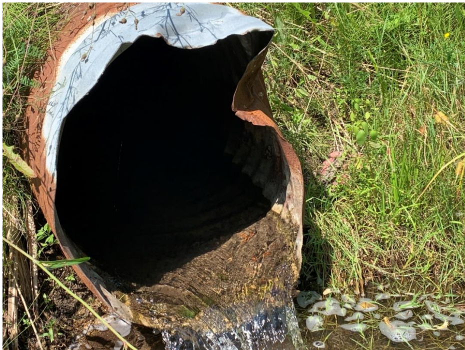
Photograph 6: Entrance at one of the twin existing CSP culvert at outlet side – August 9, 2023 (taken by EXP)
