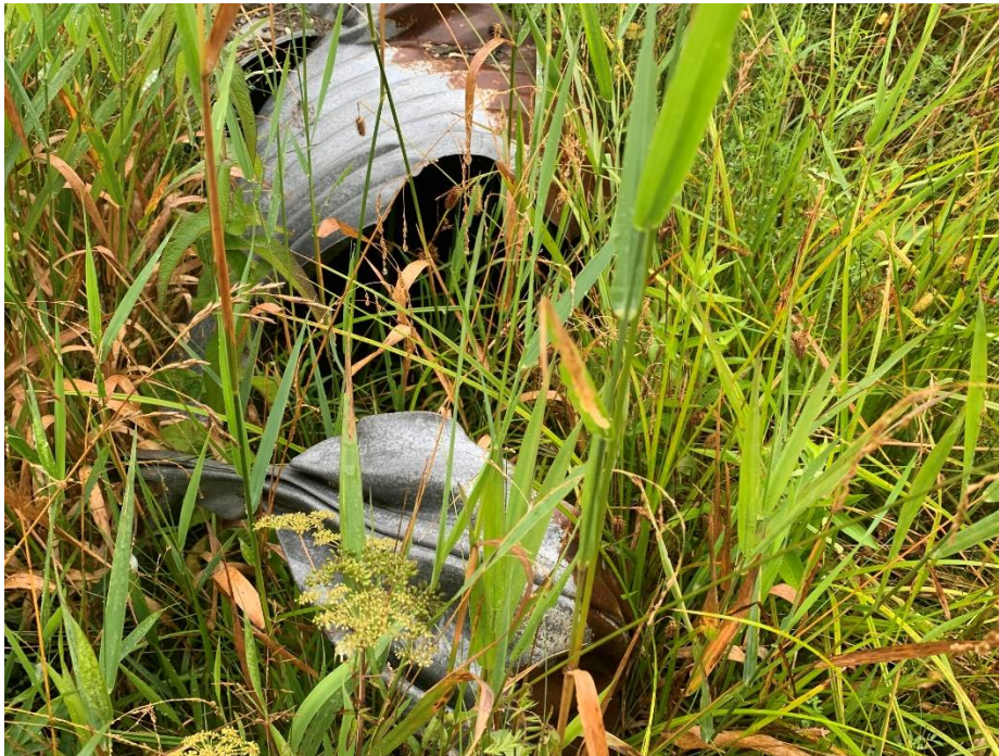
Photograph 2: Condition of one of the twin existing CSP culvert at inlet side – August 10, 2023 (taken by EXP)
