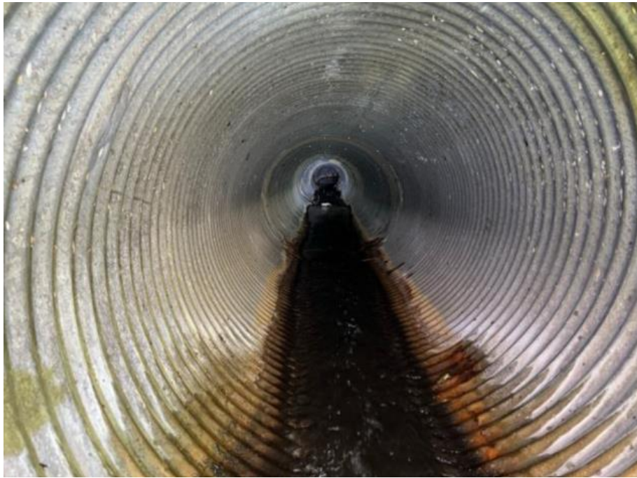
Photograph 1: Inside of existing CSP culvert at inlet side (taken by MTO)
