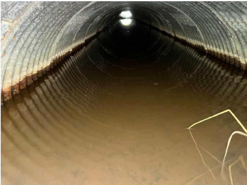
Photograph 2. Inside of existing CSPA culvert at outlet side (taken by MTO)
