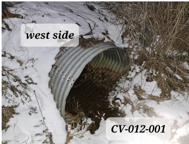
Photograph 3. Culvert inlet and embankment side slope area (facing east), January 2023 (taken by EXP)
