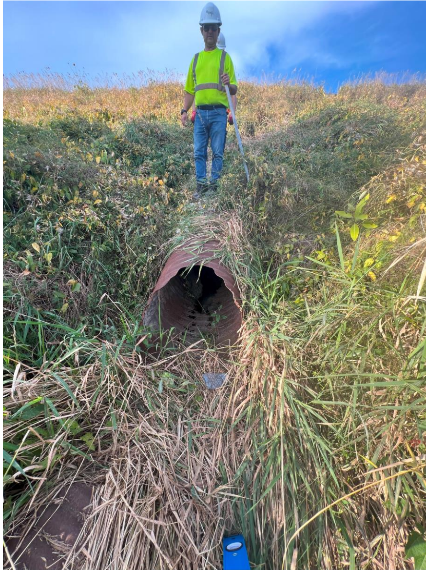
Photograph 1: Looking Northeast -Front view of existing CSP culvert at outlet side – September 06, 2023
