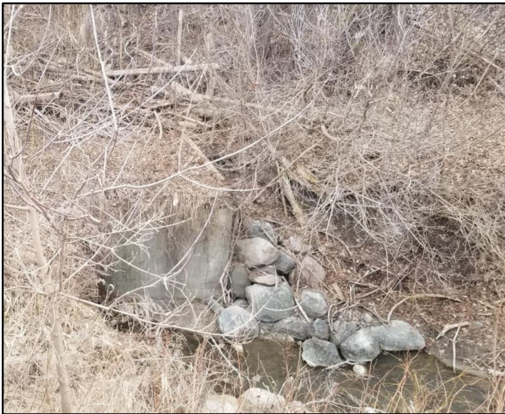
Photograph 3 – North culvert inlet, looking north (erosion near south/east side of culvert not shown) (Spring 2024)
